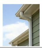
Professionally installed downspouts to direct rain water from the roof to the ground away from the building's foundation so that no rainwater is able to pool around the building. Without perfectly working downspouts, rainwater will fall off the roofs edge and may cause flooding and damage by passing through the cracks in the walls, windows and into the buildings foundation.
